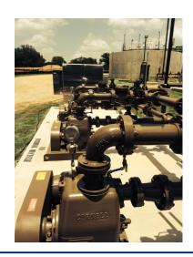
6STX Self-Priming Trash Pump Sewage and Industrial Wastewater Handling Max. 375 m<sup>3</sup>/hour, Max. 50 mwc
